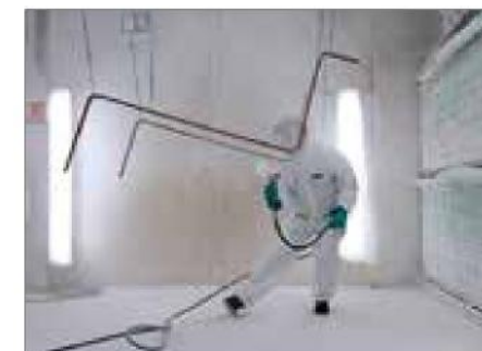
▲ The moulded wood features are painted in a booth, and this is definitely worth writing home about.
